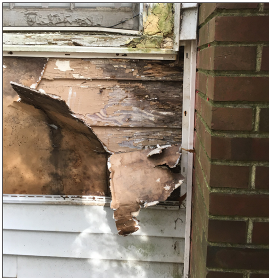
When vinyl siding was removed during renovation, wood siding was discovered underneath.
