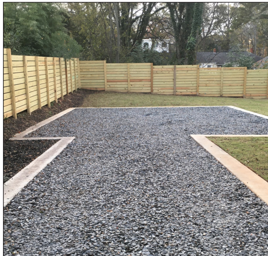
This pea gravel driveway is contained by the concrete edging, giving a more polished appearance.
