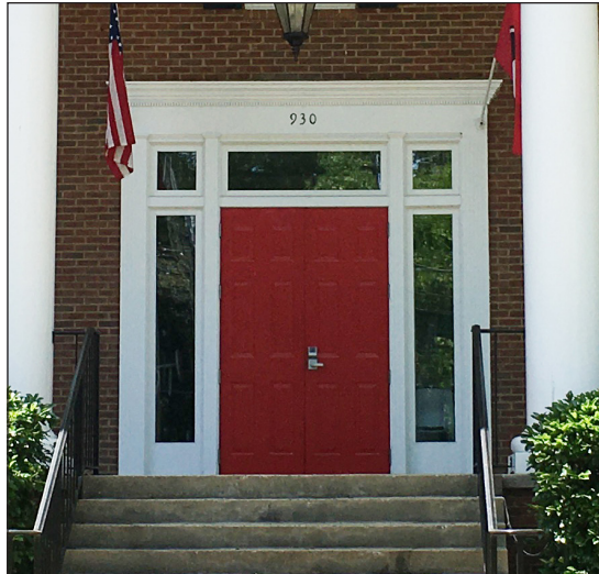
These examples show both a historic and non-historic structure having an entrance with a transom above and sidelights at each side.
