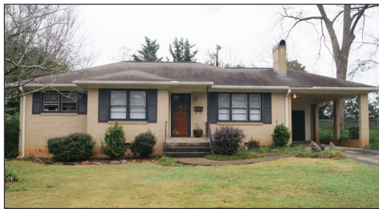
This is an example of low roof pitch. Low pitched roofs are common to Craftsman and Greek Revival styles of architecture.
