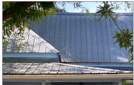
Metal roofs have become increasingly popular. However, they are not all the same. When choosing a product, look at the height of the seams, the spacing of the seams, the ridges, the finish, and the fasteners. These factors contribute to the character of the metal roofing and its appropriateness for a property.
