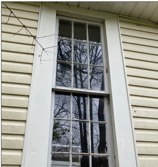
One of the problems with vinyl and aluminum siding is the loss of trim details such as the depth around window trim.
