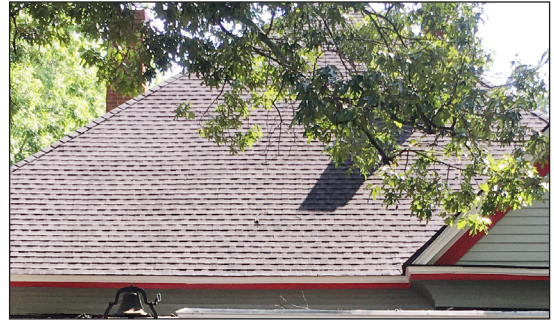
Asphalt and architectural shingles are the most common roofing materials used today.
