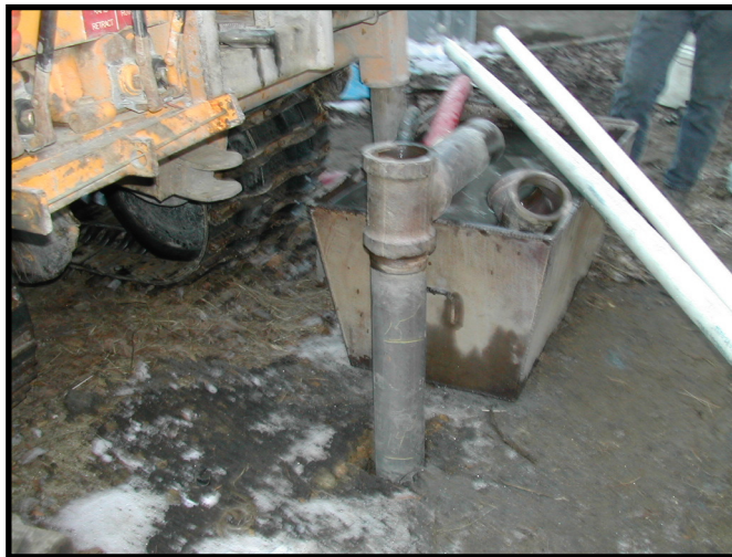
Boring holes to test for ground contamination
