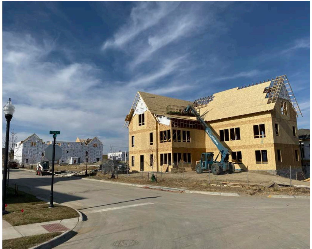
Figure 2.4 The simple forms, smaller size, and compatibility with Type V construction help maximize affordability and investment returns, and are consistent with the construction strategies familiar to most residential homebuilders, as shown in this under-construction MMH project in Papillion, Nebraska.
