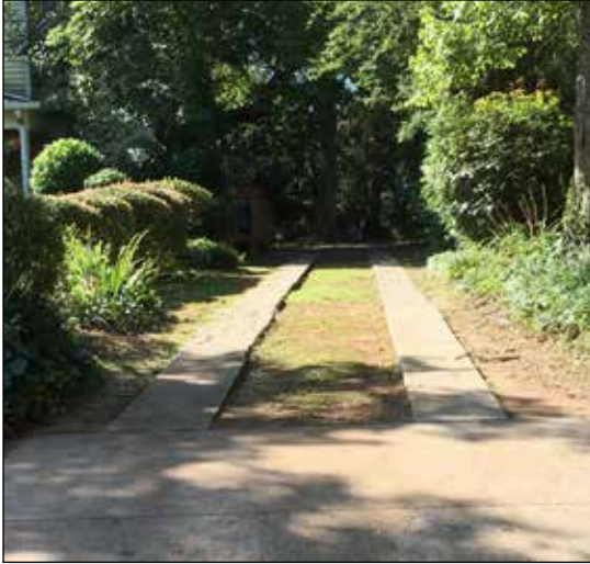
Concrete paving strips allow a grassy strip to remain and lessen the amount of paving material used.
