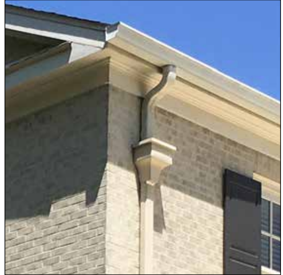
A downspout extends from an attached gutter.
