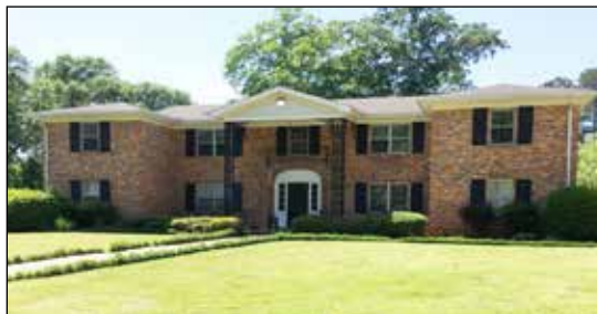
This is an example of low roof pitch. Low pitched roofs are common to Craftsman and Greek Revival styles of architecture.
