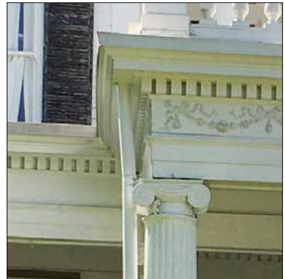
A downspout extends from a built-in gutter.
