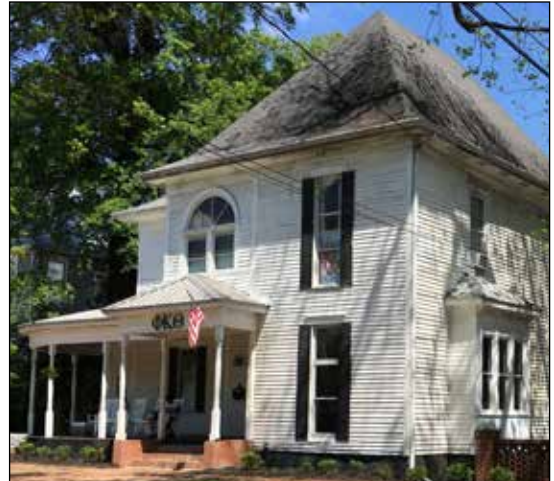
Standing seam metal roofs are more common to porch roofs than main roofs along Milledge Avenue. In this example, asphalt shingles are used for the main roof with standing seam metal on the porch.
