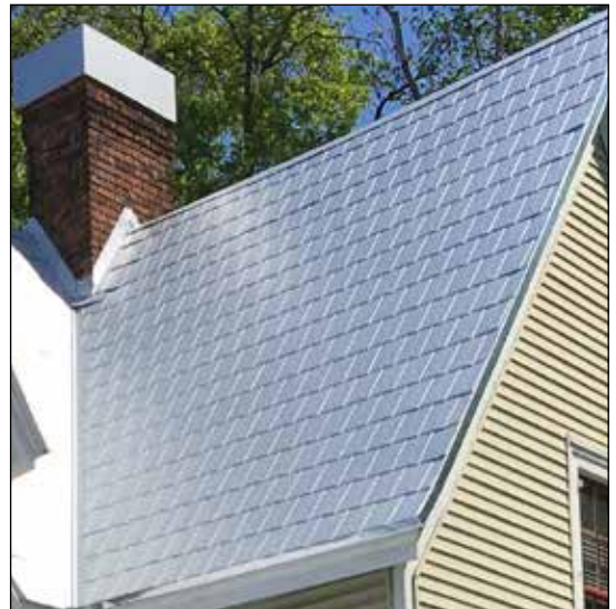
Metal shingles are found on a number of properties along Milledge Avenue. This example has a pressed pattern in each shingle.
