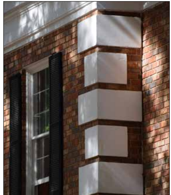
Masonry structures do not have corner boards but some examples have quoins, which are similarly situated at the corners.
