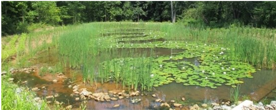
The Stormwater Management Program recognized Armentrout, Matheny, Thurmond P.C. and McLane Company in 2020 for their engineered pocket wetland, pictured above.
