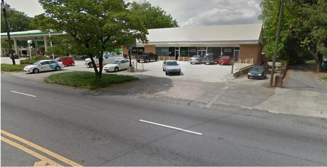
Driveways with large pan widths and undefined right-of-way and sidewalk
