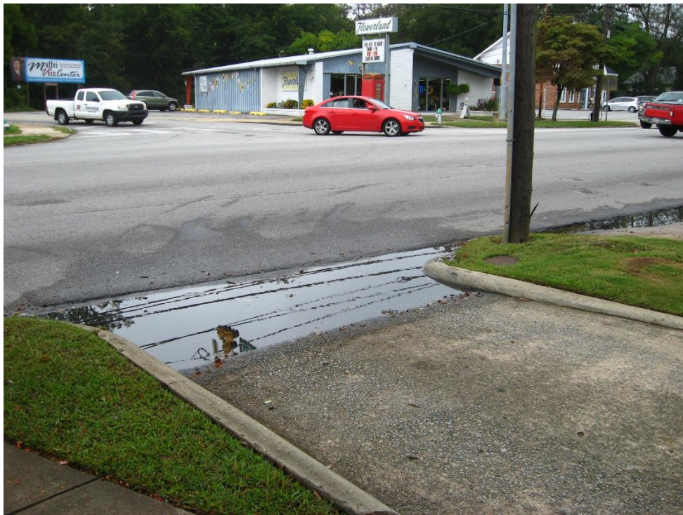
Missing drainage structure
