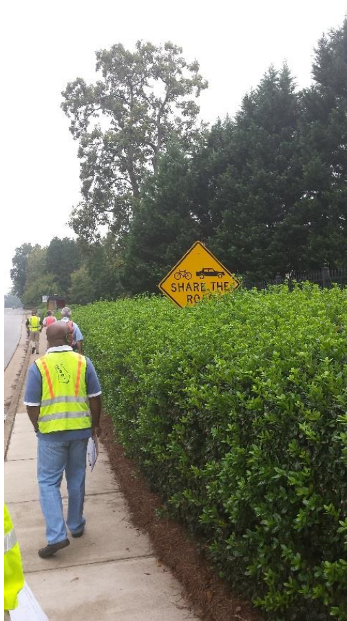
Share The Road sign is not MUTCD compliant and hidden by shrubs
