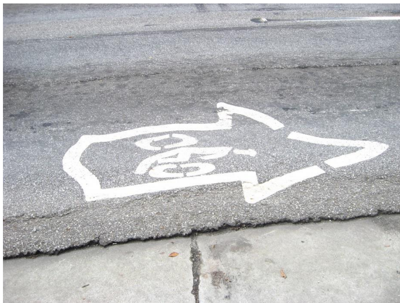
Pavement markings are not to current standards and pavement is in poor condition in some areas
