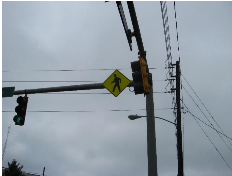
Incorrectly placed pedestrian sign at King Ave
