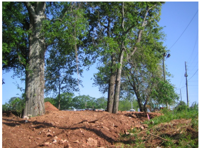
The effects of improper tree protection during tree removal and land disturbance.
