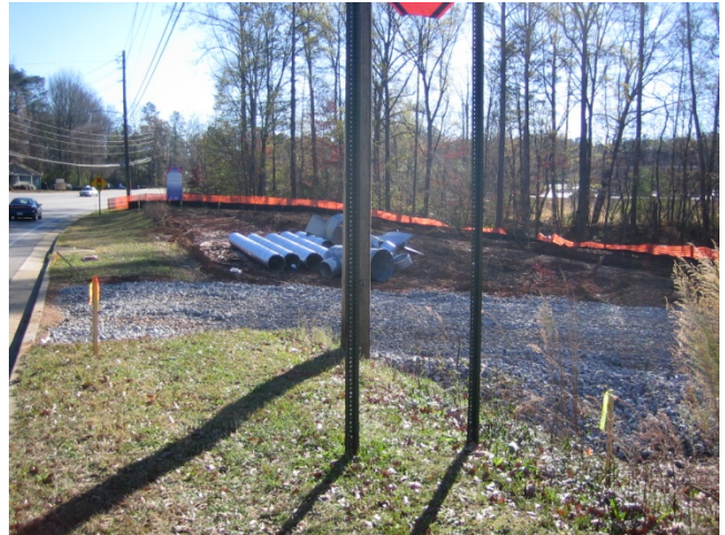
Gravel entrance to timber harvesting site – helps prevent tracking mud onto public roads.
