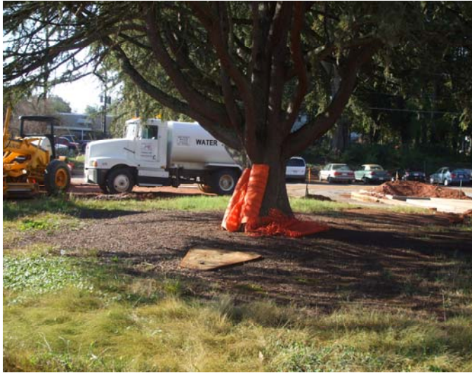
Damage is likely to occur if fencing is not installed prior to construction.
