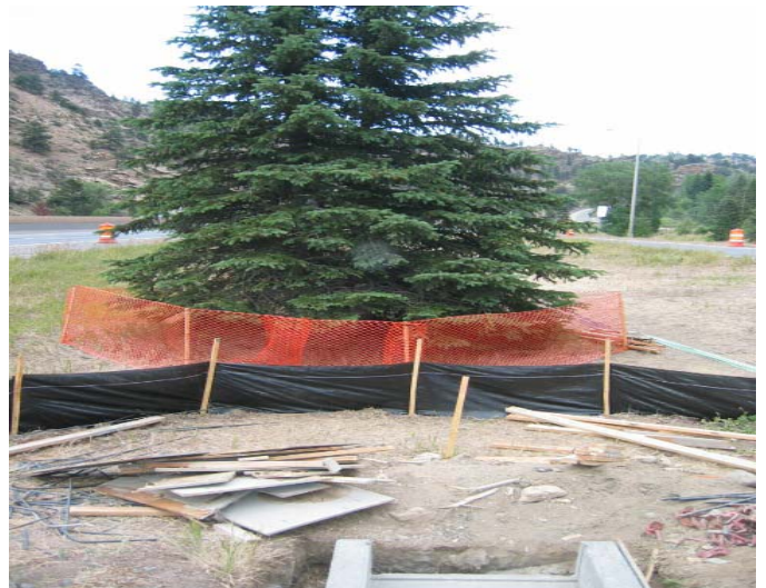
This fencing protects enough roots to ensure the survival of this tree.
