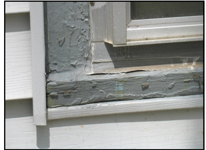
One of the problems with vinyl and aluminum siding is the loss of trim details such as the depth around window trim.
