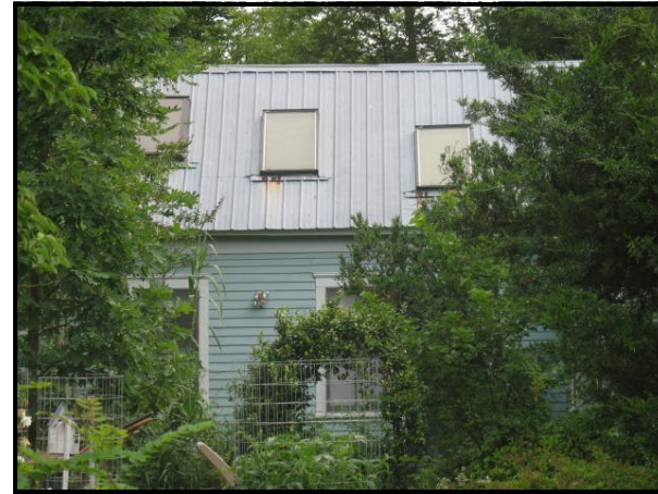
These skylights are on secondary elevations and designed to have minimal visibility from the street.
