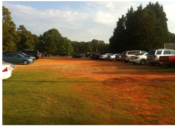
Figure A.6: Overflow parking erosion Daily use of overflow parking contributes to erosion.
