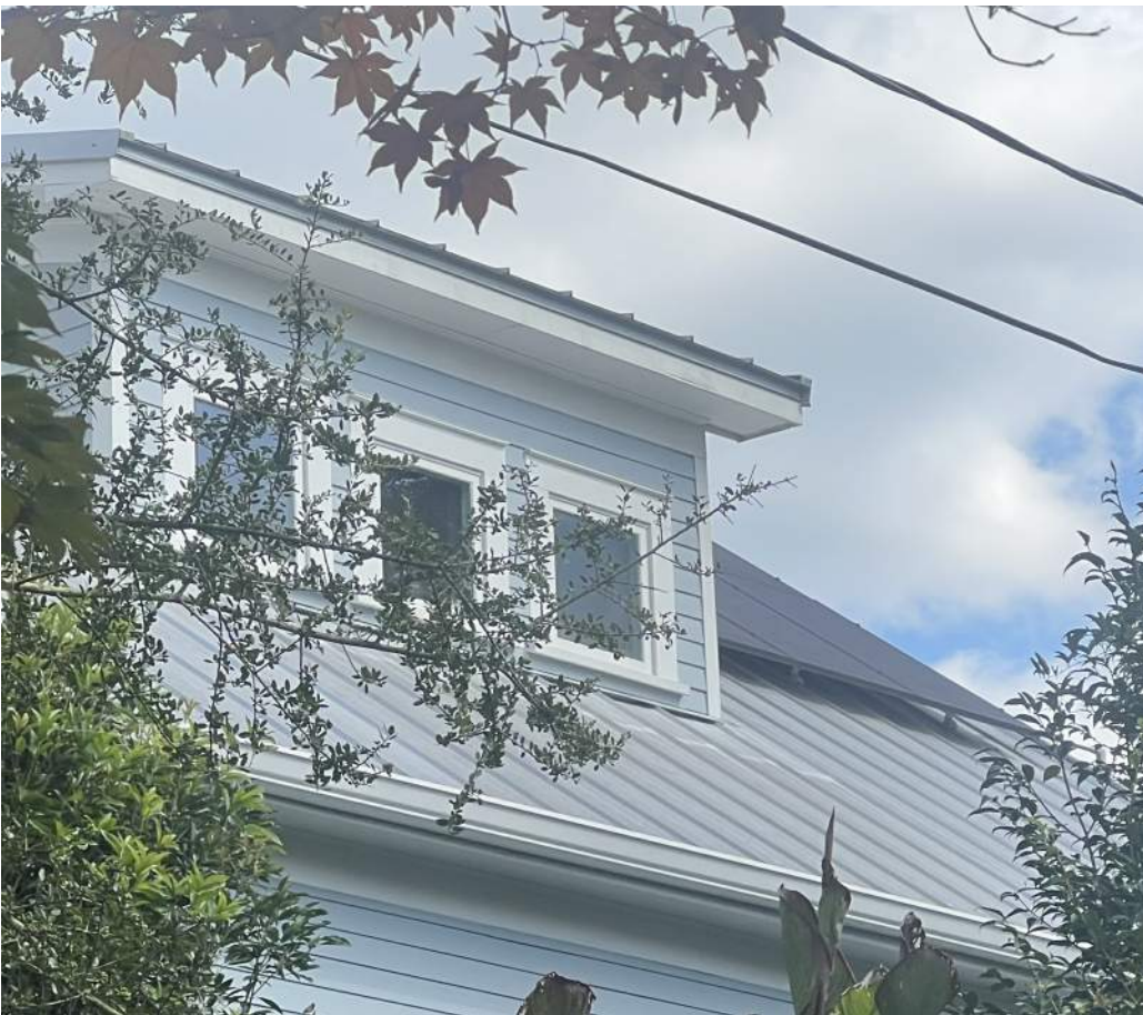
815 Blvd Solar Panels - View from Blvd
