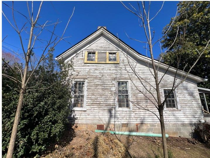
Windows exposed to weather, not covered by porch. substantial window frame deterioration, and water intrusion risk.
