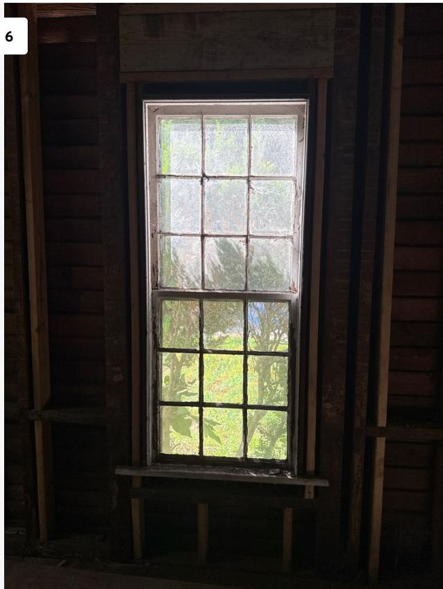
previous framing repair prevents counterweights from being installed to restore operation of existing sashes.
