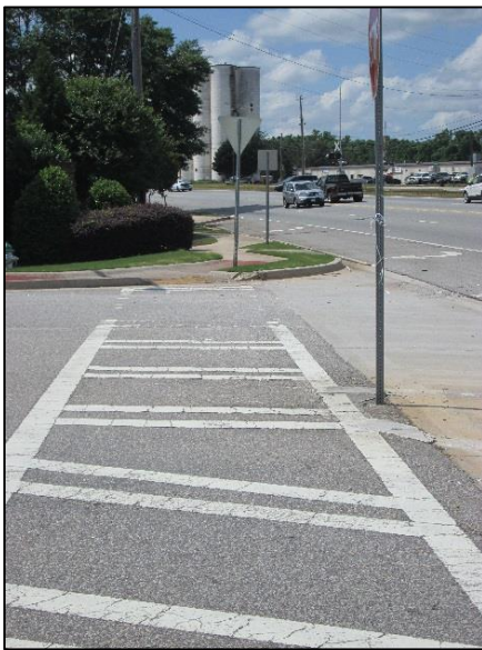
FIGURE 41. LIMITED SIGHT DISTANCE FROM PUTTERS DRIVE.
