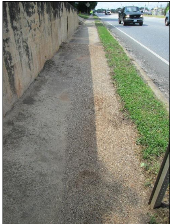
FIGURE 47. CLOSE-UP OF SEDIMENT FROM RETAINING WALL ON THE SIDEWALK.
