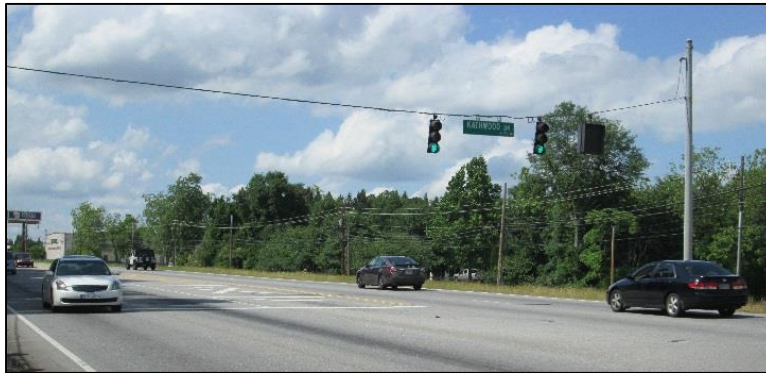
FIGURE 53. LOW-HANGING TRAFFIC SIGNALS AT KATHWOOD DRIVE.
