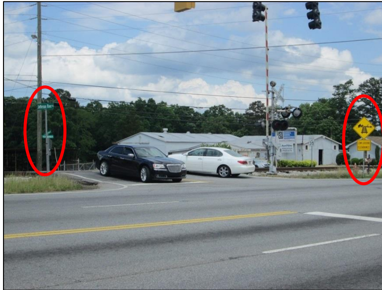
FIGURE 35. RAILROAD CROSSING AT JEFFERSON RIVER ROAD. NOTE "LOW GROUND CLEARANCE" SIGN ON FAR SIDE OF INTERSECTION AND SMALL POST-MOUNTED STREET NAME SIGN.
