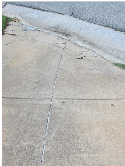
FIGURE 15. MISSING TRUNCATED DOMES ON PEDESTRIAN RAMPS
