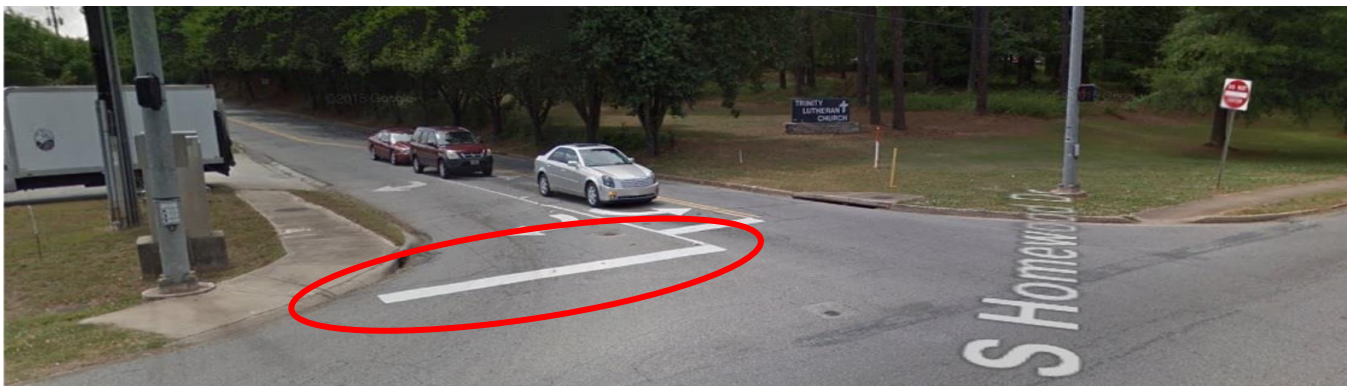
FIGURE 61. PEDESTRIAN RAMPS DO NOT ALIGN AND STOP BAR IS AHEAD OF PEDESTRIAN RAMP ON SOUTHWEST CORNER.
