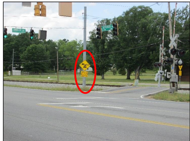
FIGURE 26. LOW GROUND CLEARANCE SIGN ON FAR SIDE OF INTERSECTION SHOULD BE RELOCATED TO NEAR SIDE.
