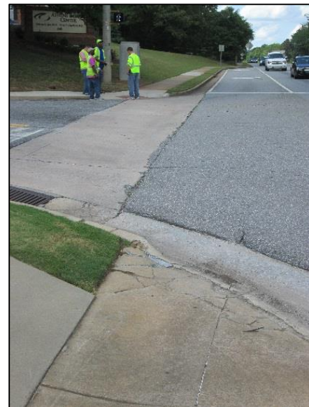
FIGURE 56. SIDEWALKS INCORRECTLY ALIGNED FORCE PEOPLE ON THE SIDEWALK INTO TRAVEL LANES.
