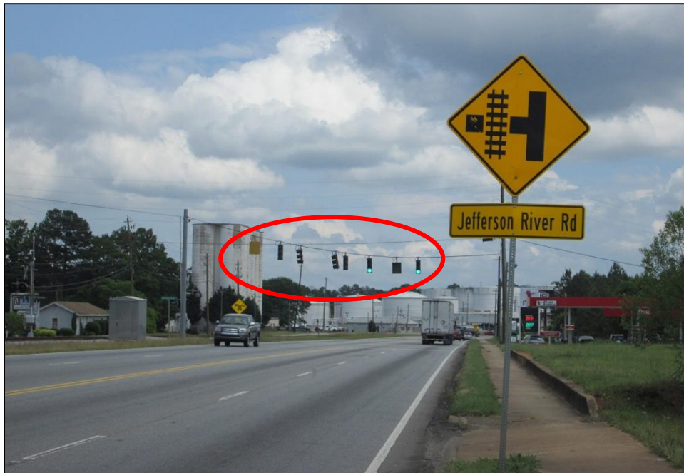
FIGURE 34. JEFFERSON RIVER ROAD INTERSECTION, VIEWED FROM SOUTHBOUND LANES. NOTE ALL TRAFFIC SIGNALS ARE ON SAME OVERHEAD LINE.
