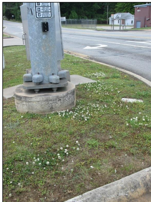
FIGURE 16. OUTDATED PEDESTRIAN SIGNAL PUSH BUTTON WITH NO PEDESTRIAN RAMP OR SIDEWALK.
