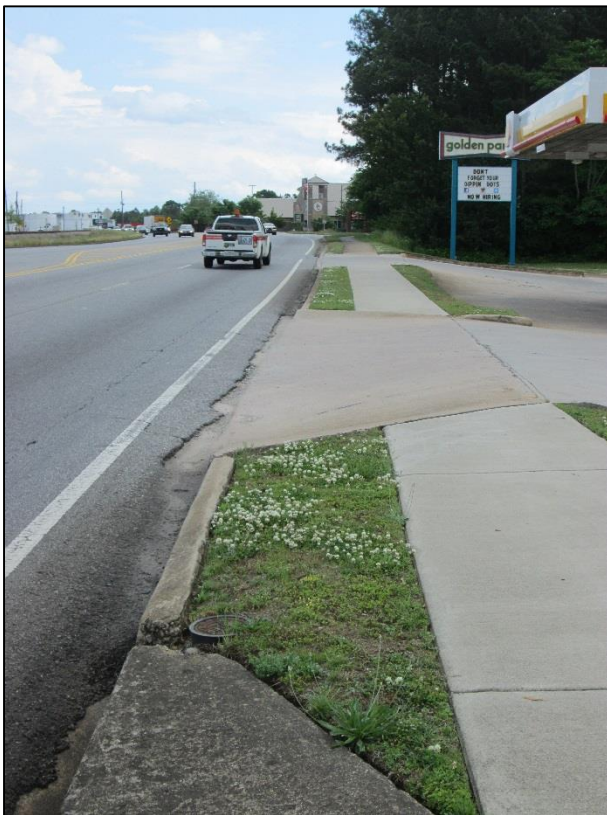
FIGURE 25. DRIVEWAY TOO CLOSE TO INTERSECTION AND NO LEFT-TURN LANE INTO GAS STATION.
