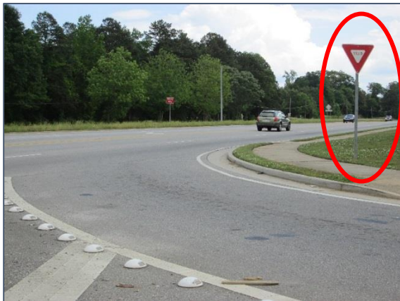
FIGURE 22. YIELD SIGN AT INCORRECT ANGLE IN THE SOUTHWEST CORNER OF THE INTERSECTION.
