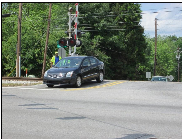
FIGURE 12. SINGLE VEHICLE FILLS STORAGE AREA BEHIND STOP BAR ON JEFFERSON RIVER ROAD.
