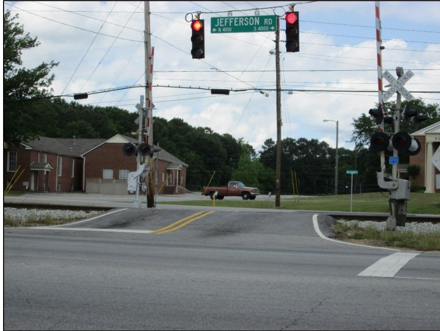
FIGURE 28. RELATIVELY STEEP GRADE AT RAILROAD CROSSING ON WHITEHEAD ROAD.
