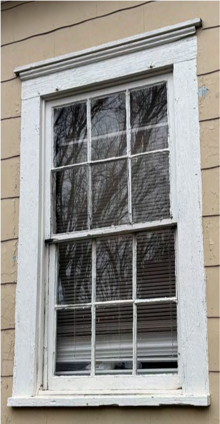
WINDOW B WOOD WINDOW ROT, FALLING APART
