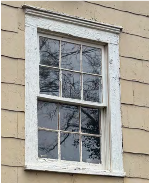
WINDOW A WOOD WINDOW ROT, DEGRADED
