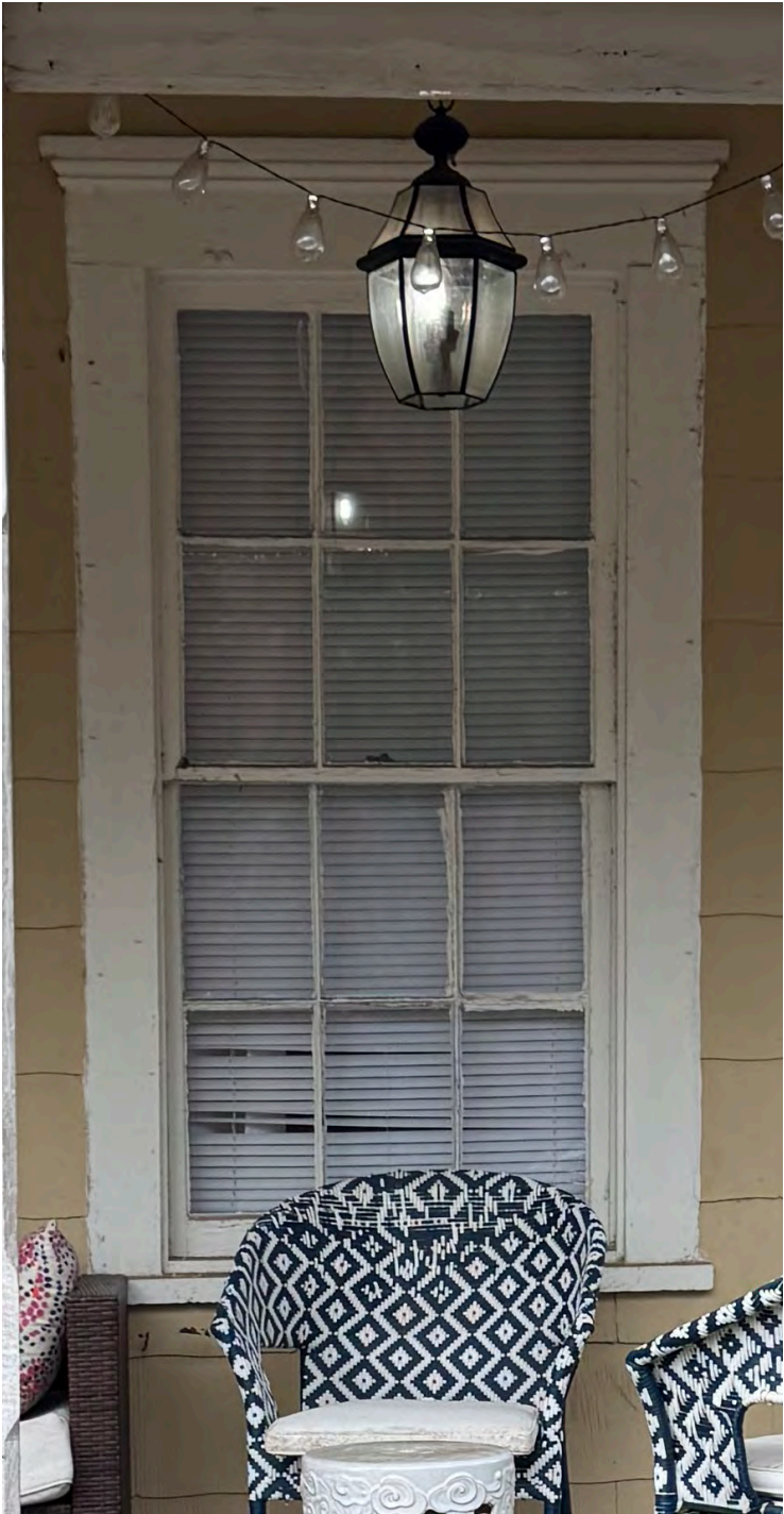
WINDOW B WOOD WINDOW SIGNS OF ROT
