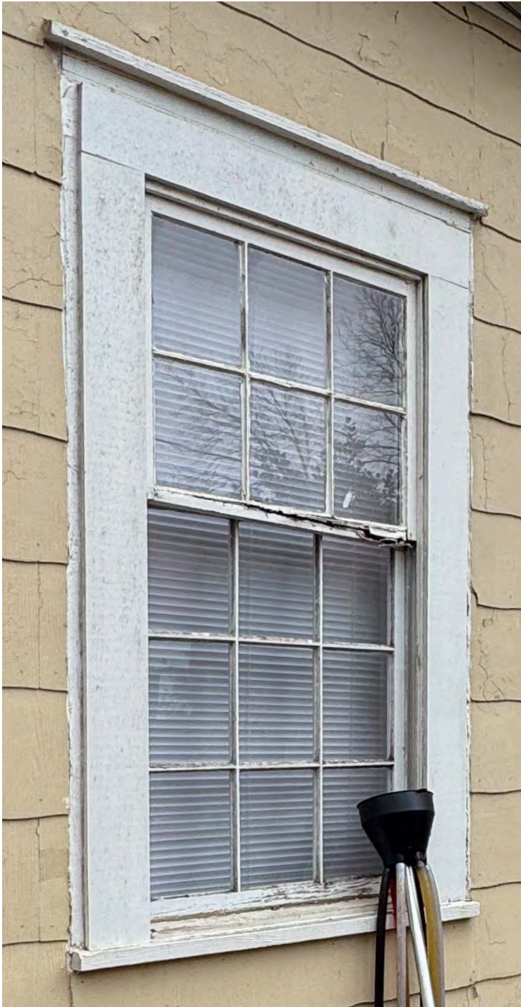
WINDOW A WOOD WINDOW ROT, FALLING APART
