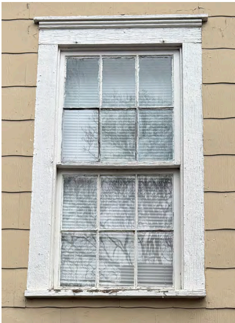
WINDOW A WOOD WINDOW ROT, IRREGULAR REPAIRS
