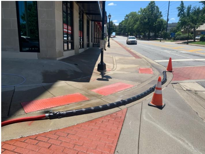
During a power washing project at The Standard, a wastewater containment system similar to the Vacu-Boom was used to capture all runoff effectively. The system created a seal around the work area, ensuring that no washwater entered storm drains or surrounding areas.
